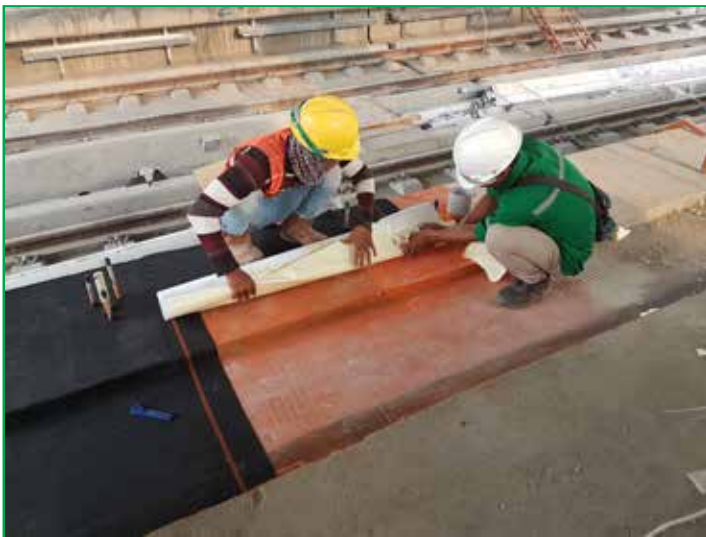
APPLYING M-SEAL® VM500 ONTO STATION PLATFORM SLAB
