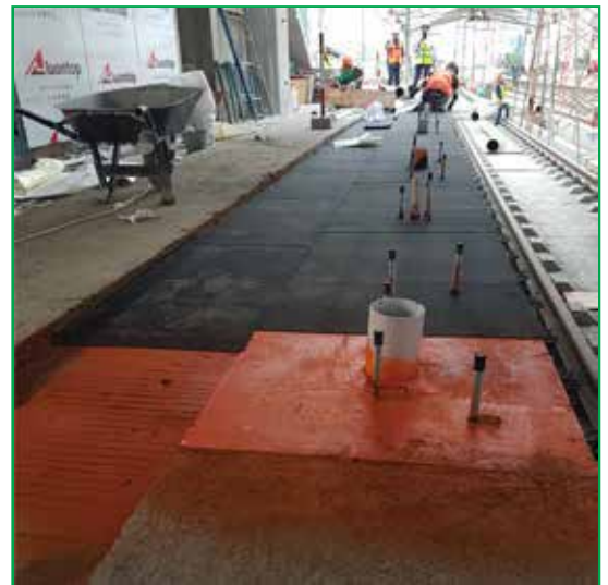
APPLYING M-SEAL® VM500 ONTO STATION PLATFORM SLAB
